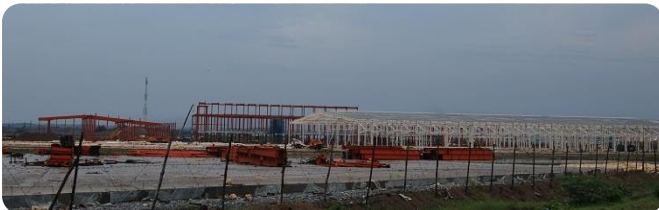
SAIC GM Wuling Construction Progress
