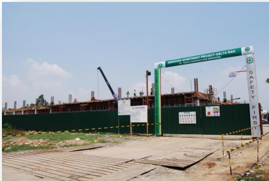
Serviced Apartment Construction Progress as of November 2015
