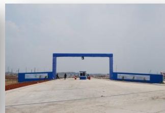
SAIC GM Wuling Construction Entrance
