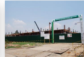
Serviced Apartment Construction Progress as of Nov 2015
