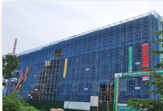
Serviced Apartment Construction Progress as of February 2016
