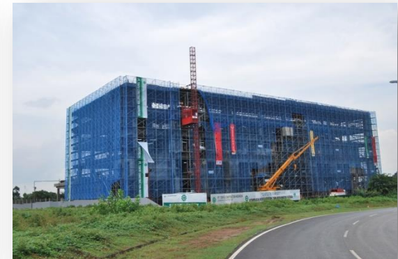
Serviced Apartment Construction Progress as of February 2016 (different angle)
